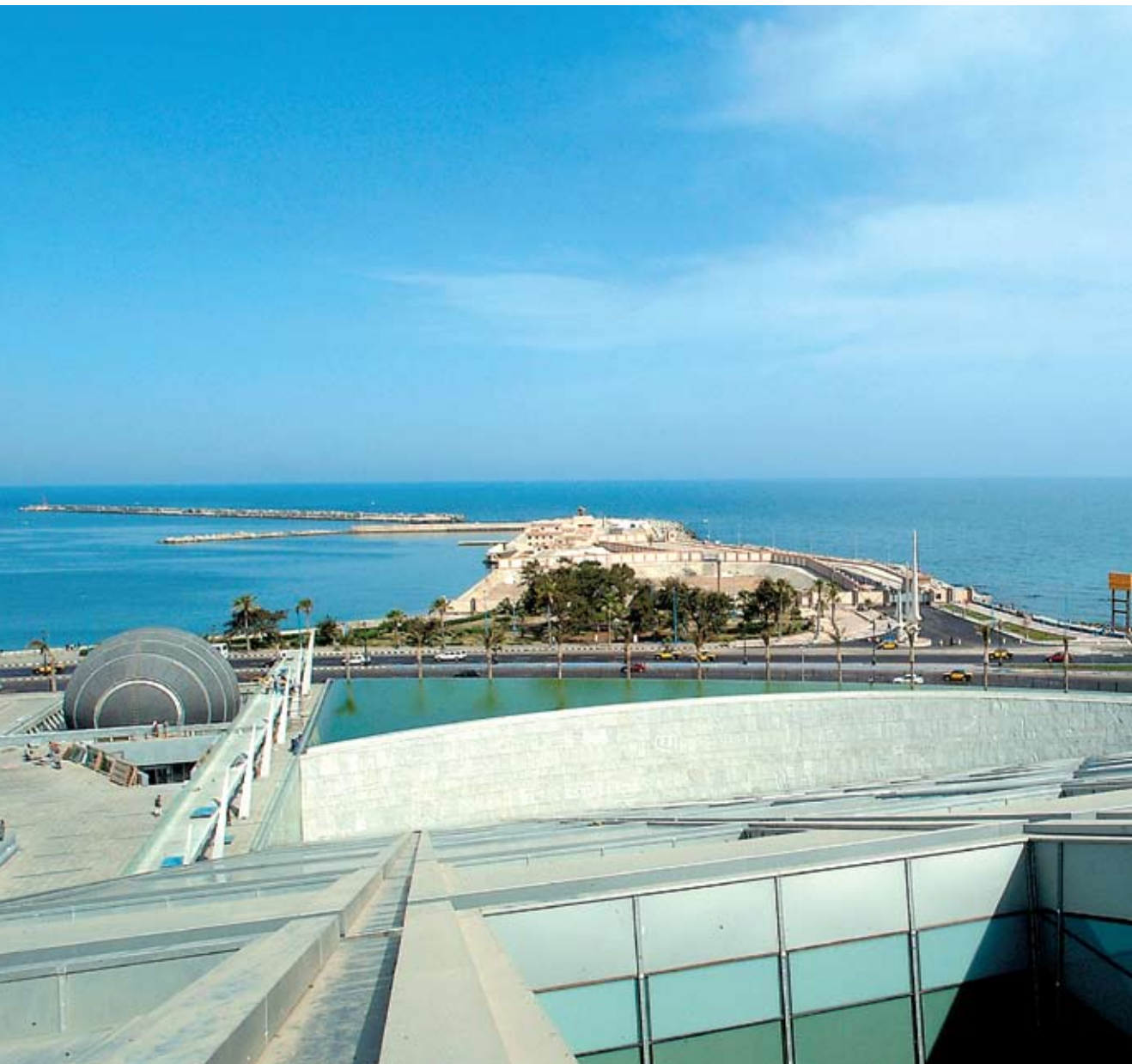
Looking out from over the roof of the Library at the Silsilah and the sea
